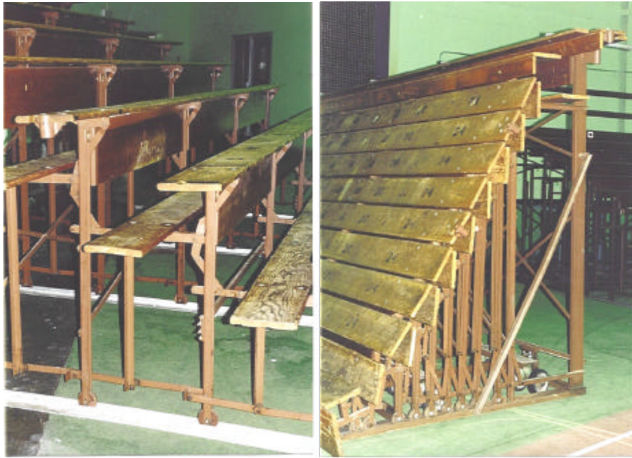
Figure 3: Telescopic bleachers (open and closed positions)
